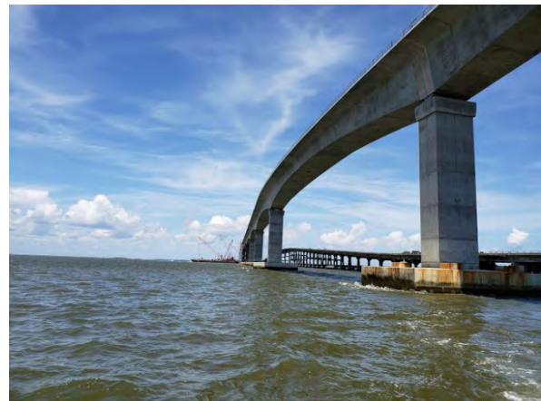
Figure 16 Bonner Bridge (high value bridge)
