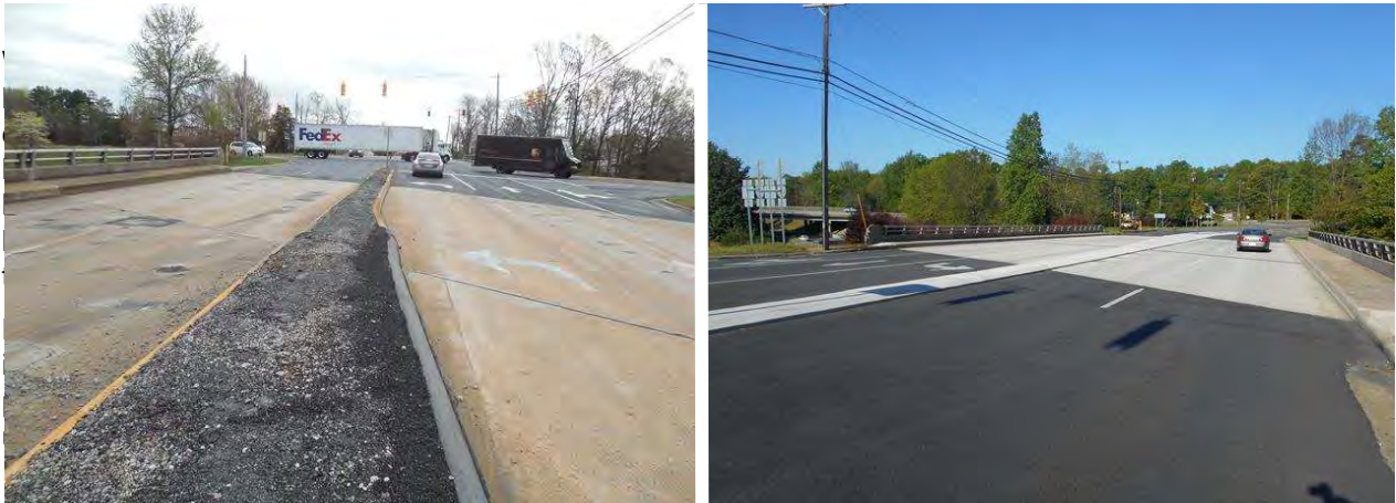
Figure 18 Damaged and Repaired Bridge Deck
