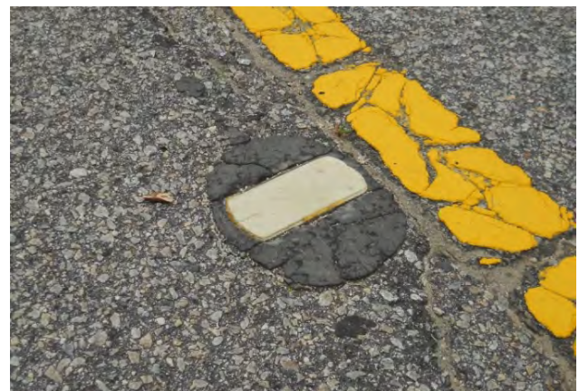
Figure 20 Damaged Pavement Markers
