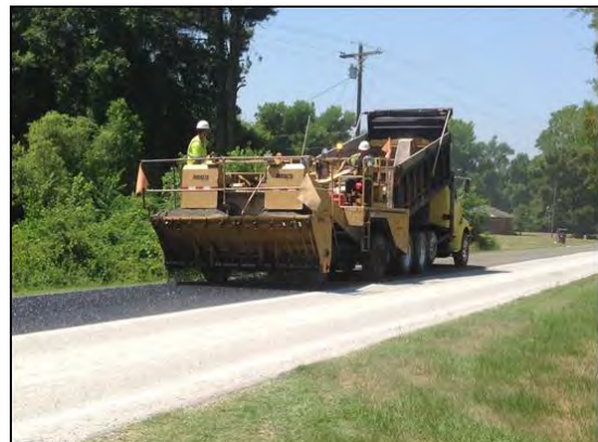
Figure 6 Pavement Preservation (chip seal)
