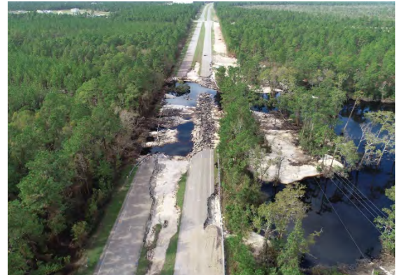
Figure 2 Hurricane Florence Damage US 421
