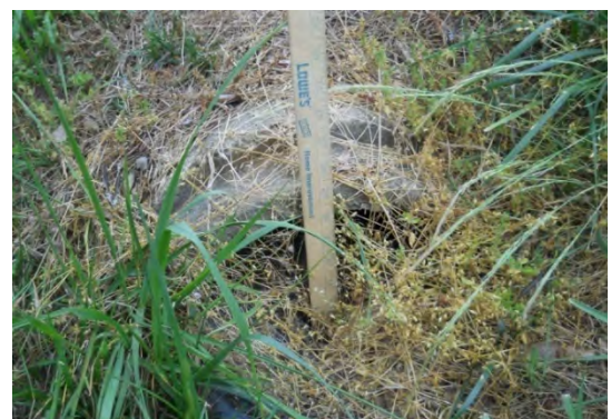
Figure 19 Blocked Crossline Pipe
